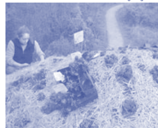
Planting the green roof
