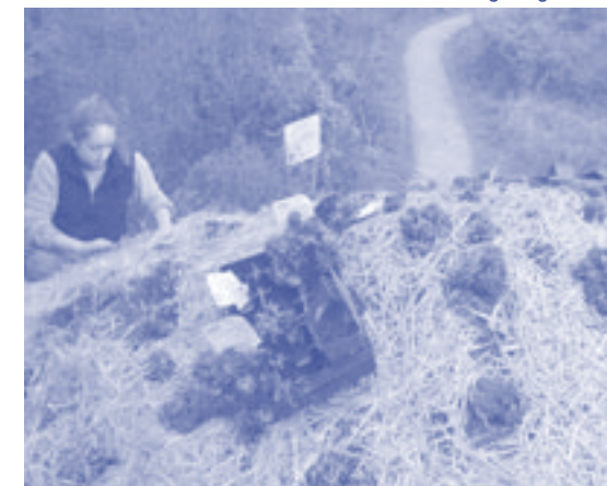
Planting the green roof
